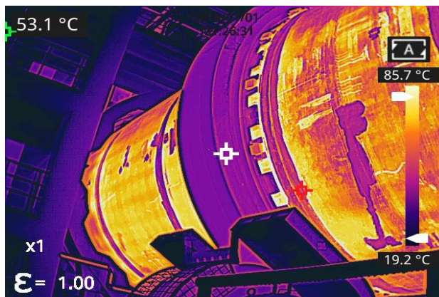
Figure 7.4 Defect Detecting of Refractory Material in Rotary Kiln
